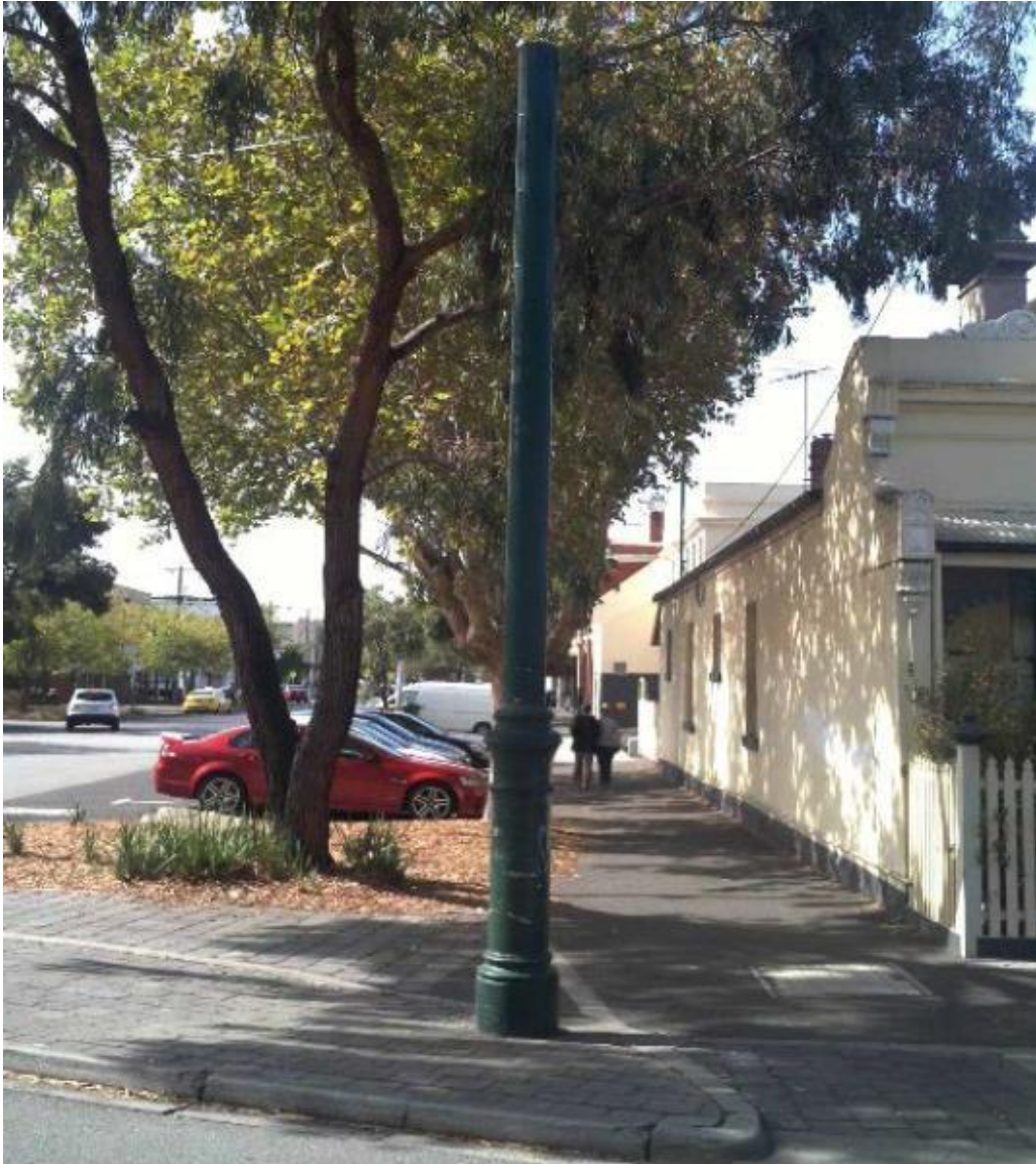
Figure 13: Sewer vent shaft
